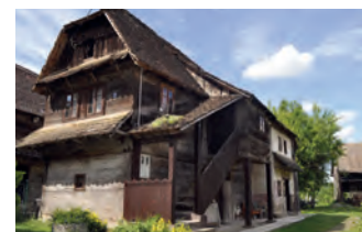
Tradicijska drvena gradnja Posavine, Lonjsko polje | Traditional wooden architecture of Posavina, Lonjsko polje Nature Park
